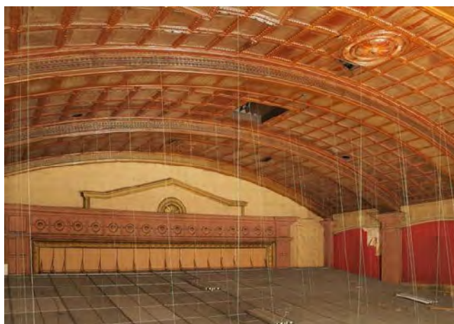
The barrel vaulted, pressed-metal ceiling at the Curzon Cinema in Clevedon, built 1920-22
